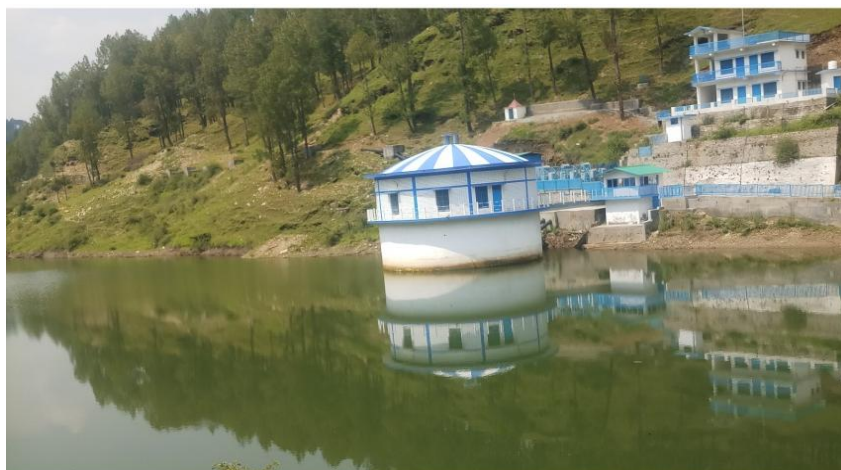
Plate 1: The Kosi drinking water pump house at Kosi which is the site for the collection of water samples
