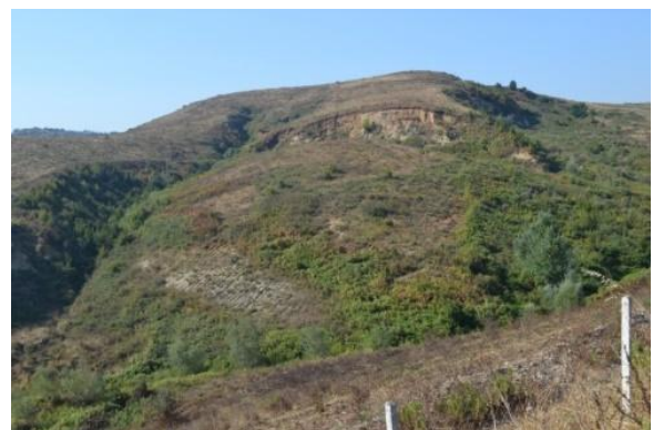
Figure 1: Examples of landslides in the study area.
