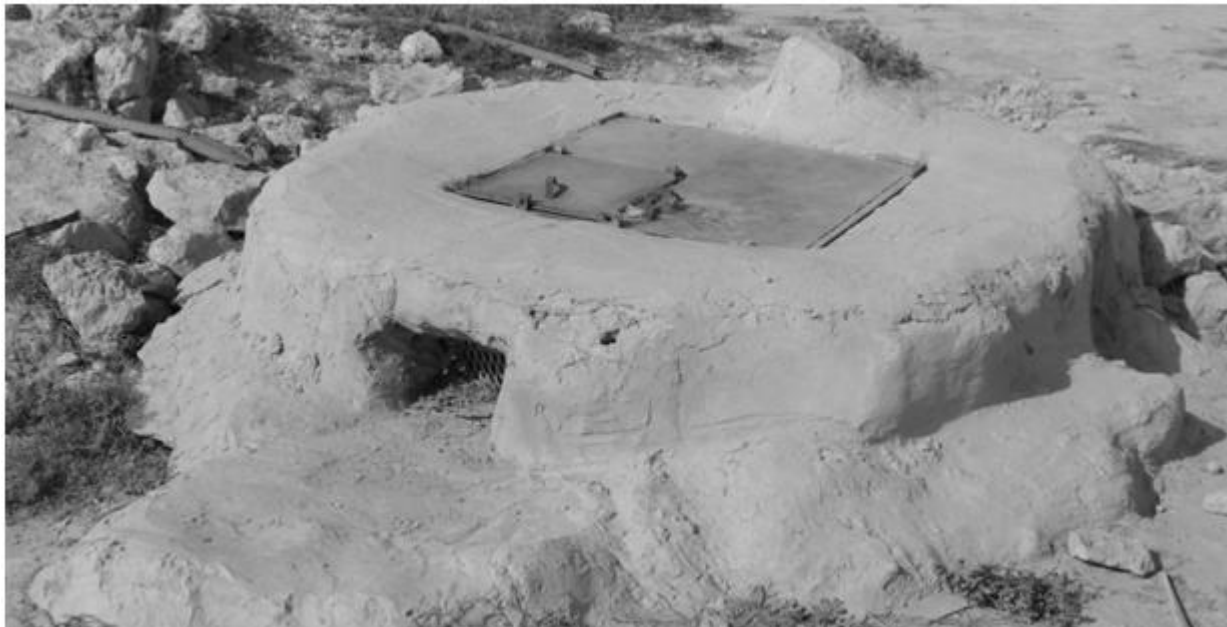
Figure 3: A Roman - style canister used for rainwater storage in a suburb area around Tobruk ( Photo by; Abdulla, 2010 ).
