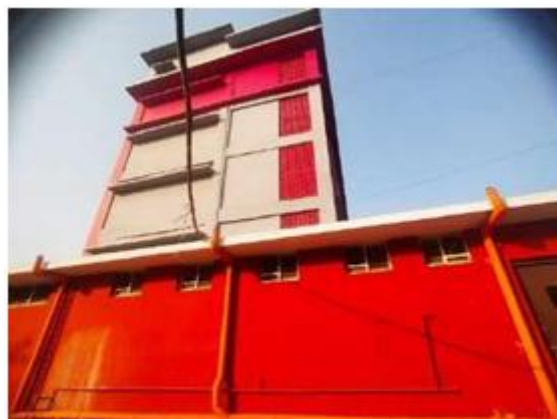
Figure 4.12: East Side Image AU-HUB Building
