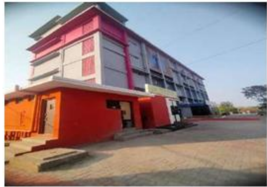
Figure 4.1: The AU-HUB Building in the Campus of the Andhra University College of Engineering, Andhra University, Visakhapatnam
