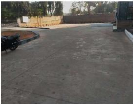
Figure 4.14: Concrete Pavement (North) (AU-HUB Building)
