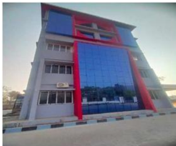
Figure 4.13: West Image (AU-HUB Building)
