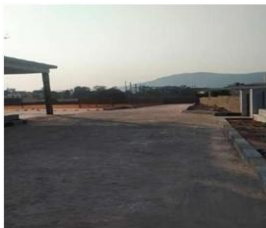
Figure 4.11: Concrete Pavement (West) Surrounding the AU-HUB Building
