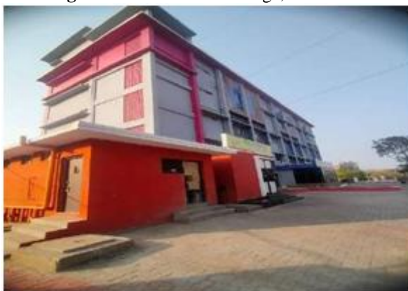
Figure 4.6: North East Image (AU-HUB Building)
