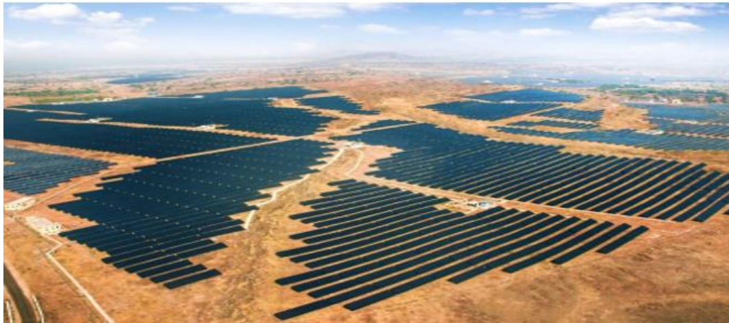
Bhadla Solar Park
