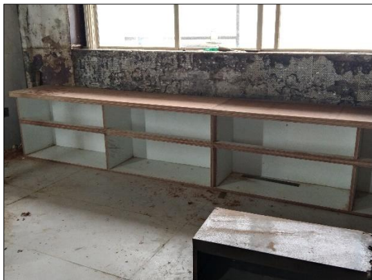
Figure 3: Condition of the Window Wall on Level 2
