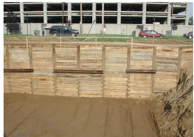
Photo 1: Tiebacks with common walers
