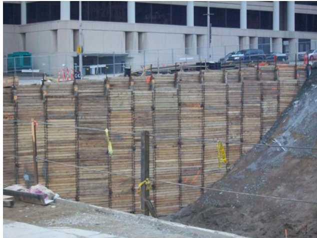
Photo 2: Tieback through pile penetration
