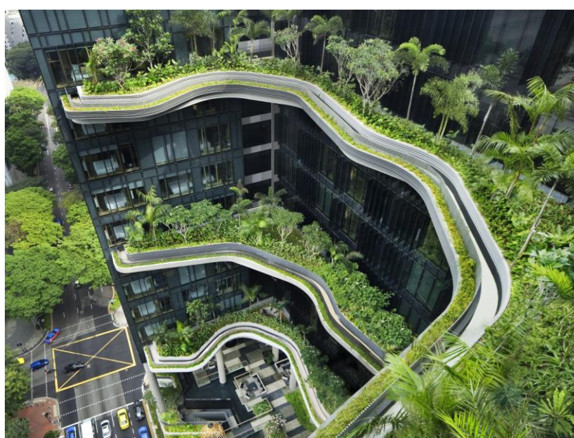
Figure 4: showing green roofs and walls (Photo Credit: WOHA / Patrick Bingham-Hall)
