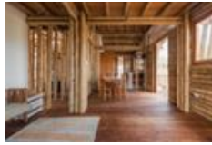
Figure: Used in columns, beams and walls
