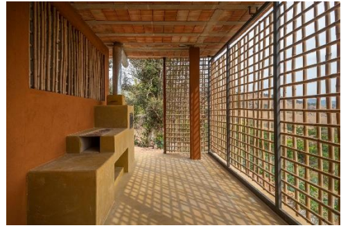
Figure: Bamboo in façade
