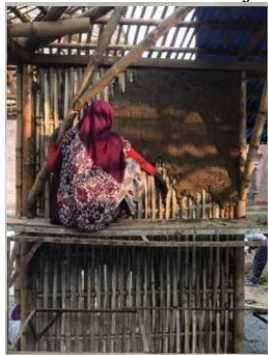
Figure: Daub walls construction
