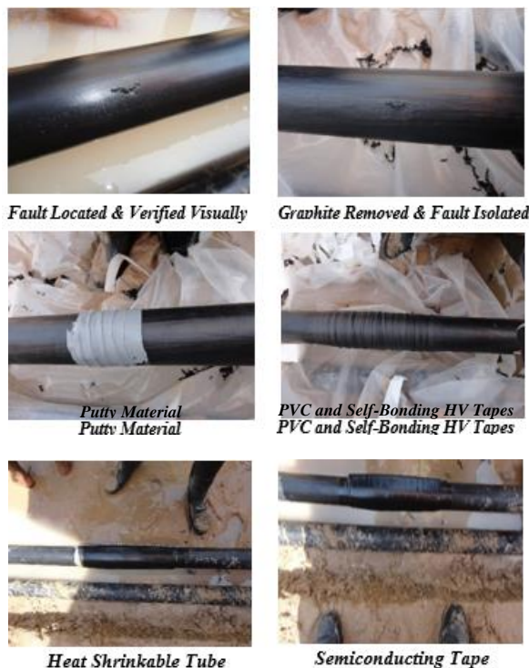
Figure 3: Sheath Fault Rectification
