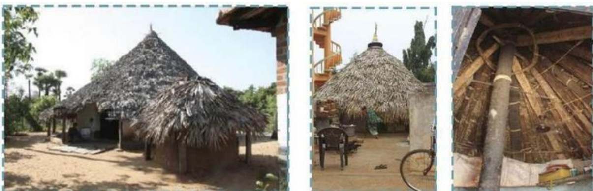
Figure 5: Typical Thatch Roof Constructions of Visakhapatnam Fishermen
