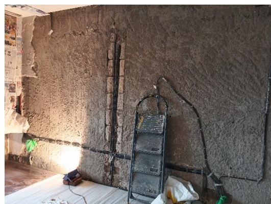
Figure 6: Work in Progress
