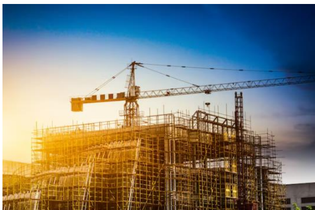
Figure 1: High rise Building construction site
