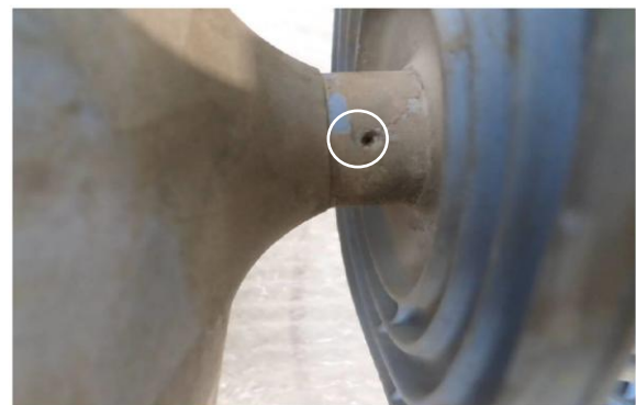
Figure 5: Defective insulator identified using DSLR Camera
