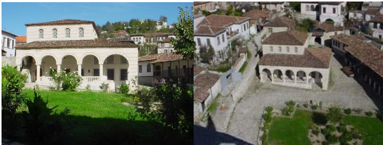
Figure 2: HelvetiMasjid, Berat, Albania. It dates back to 1492-1493. According to data next to the Small Mosque, has been linked the adjacent library. The library building was burned down during the First World War. The presence of the adjacent library tells us that the building was not only the cult object to teach the youth of the Muslim religion but also the city's school. Courtesy of Institute of Cultural Monuments of Albania.
