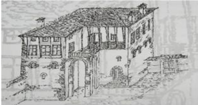
Figure 5: CENE Building , Source ICM
