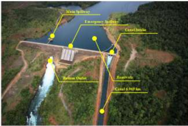
Figure 1: Aerial photograph of Batubesi Dam
