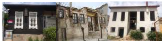
Figure 14: Suspended chimney examples in Yayla Quarter (106 Block of Buildings 4 Parcel, 728 Block of Buildings 23 Parcel, 87 Block of Buildings 8 Parcel number houses)
