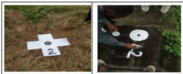
Figure 6: Establishment of Target for Ground Control
