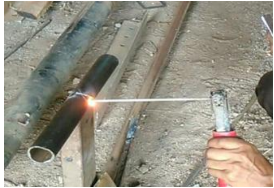
Figure 8: 5G position welding
