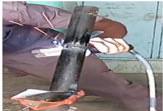
Figure 9: 6G position welding
