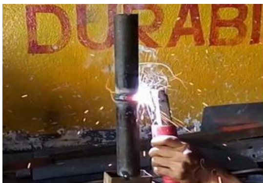
Figure 7: 2G position Welding
