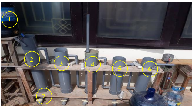
Figure 2.1: Domestic wastewater treatment system used in research (1- Inflow water tank; 2- Aerobic tank; 3, 5- Reverse filtration tank 1 and 2; 4- Anaerobic tank; 6 Inflow water storage tank 7- Sludge Flush valve)
