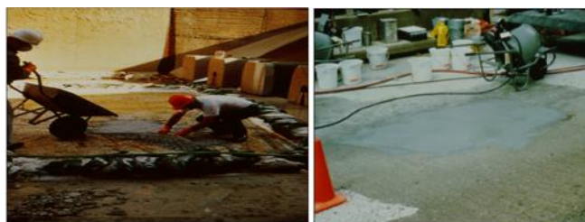
Figure 16: Placing polymers in a repair area before and after
