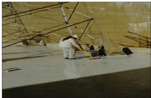
Figure 17: Overlay application with brooms, squeegees or heavy industrial grade paint roller
