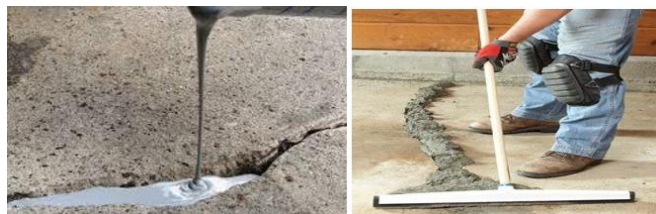
Figure 13: Gravity filling method of crack repairs
