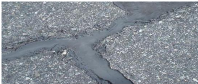
Figure 14: Dry-pack method of crack repairs
